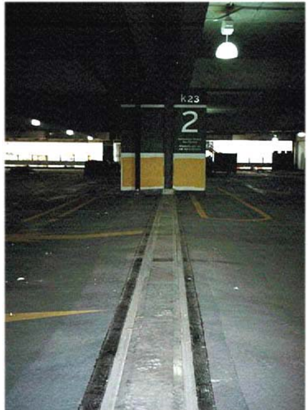
Toronto's Pearson International Airport – 30,000 feet of SSP with PyroFlex Fire Barrier
