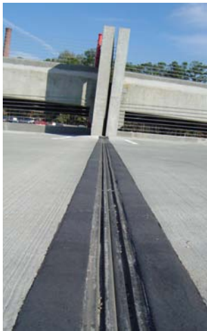
◀ example of neat workmanlike finished installation
